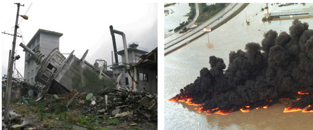
Fig. 1. Left: Collapsed structure at a fertilizer producer due to the 2008 Wenchuan earthquake in China (Photo © E. Krausmann); Right: Burning oil from a breached pipeline caused by flooding of the San Jacinto River in Houston, TX, in 1994 (Photo © U.S. Geological Survey).
