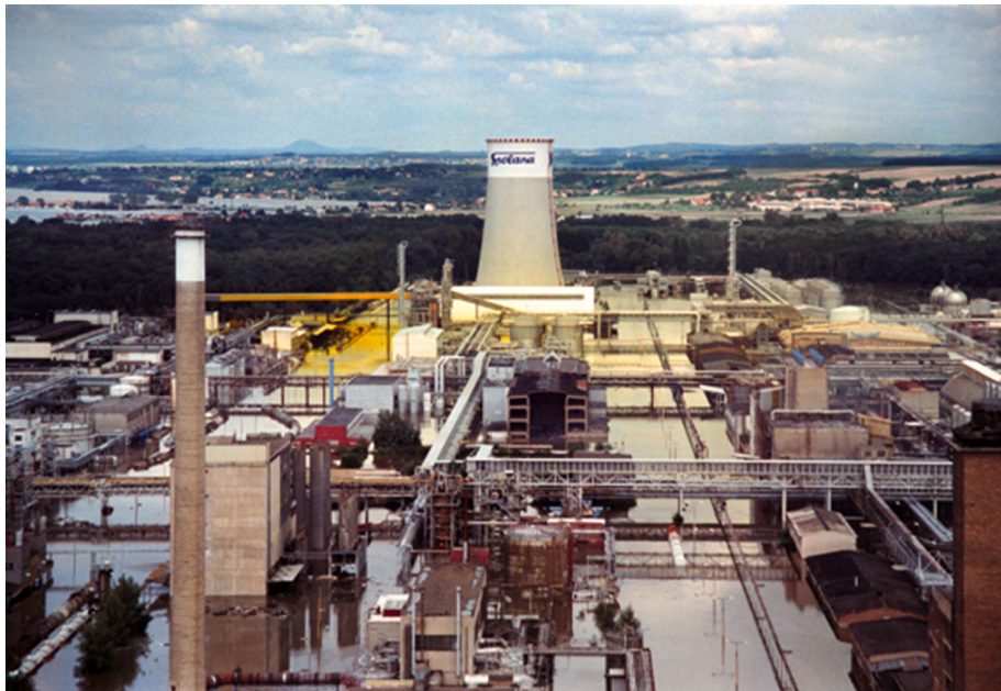
Fig. 2. Flood-triggered chlorine release (in yellow) into the air and floodwaters in the Czech Republic in 2002 (Photo © Václav Vašků). (For interpretation of the references to color in this figure legend, the reader is referred to the web version of this article.)
